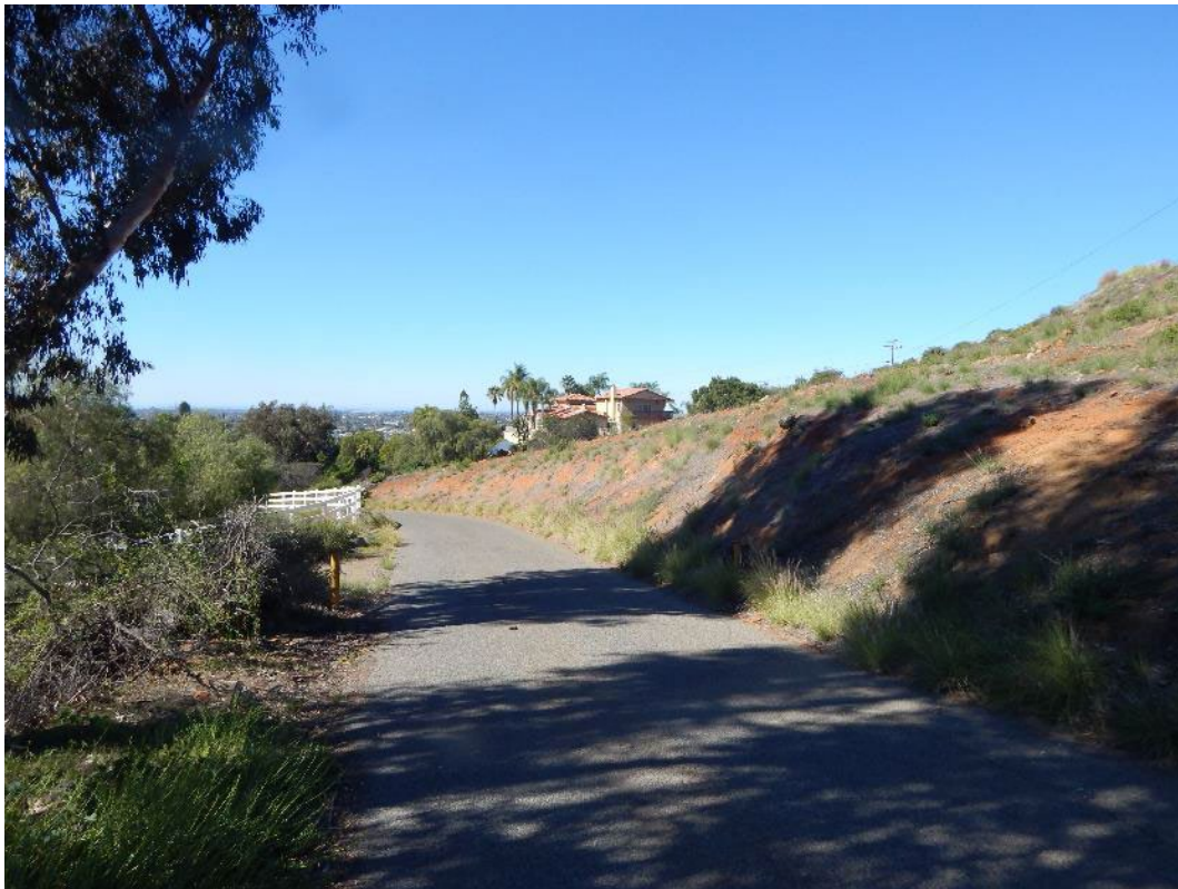
Plate 2. Overview of access road, looking west
