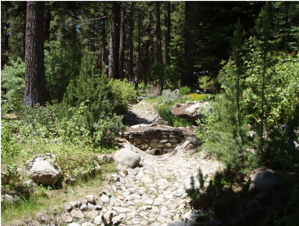
Rock lined swale surrounded by vegetation.
