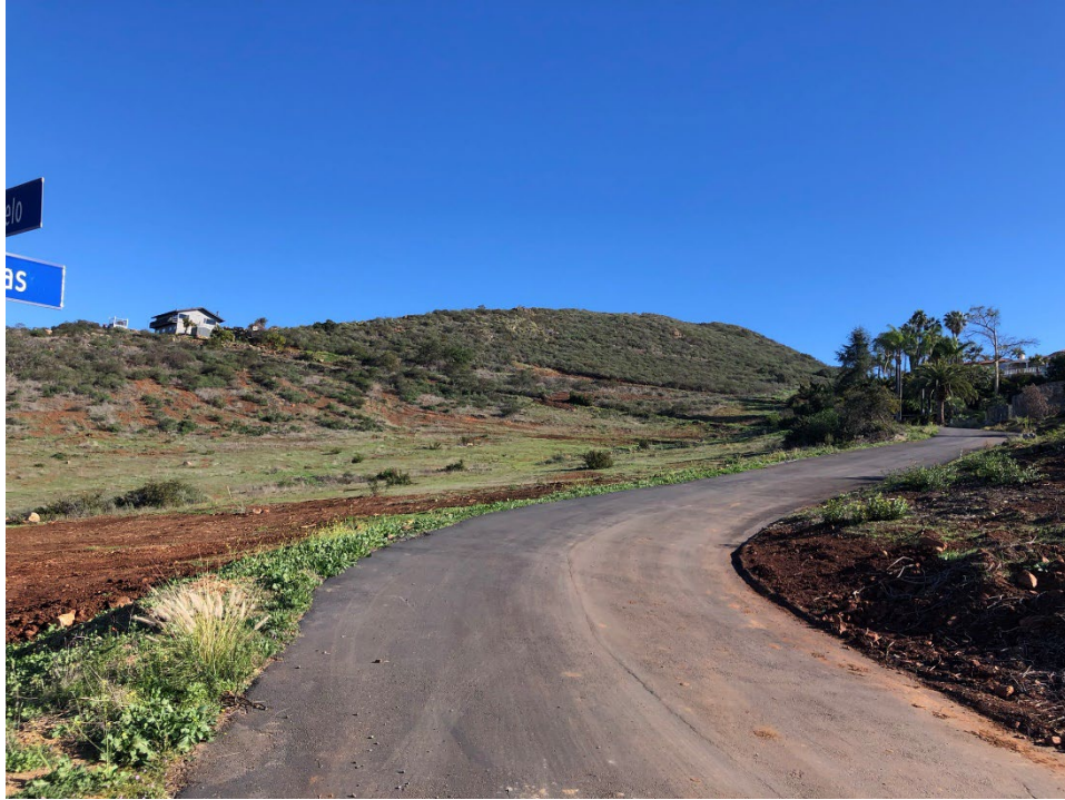
Photo 7: Looking up Las Lomas from the intersection with Tierra Del Cielo. This road will be widened into a fire access capable road up to the Canary Island palm tree at the end of the visible road in this photo. The Lot 7 parcel is on the right side of the road here and the 1985 Las Lomas parcel is on the left.
