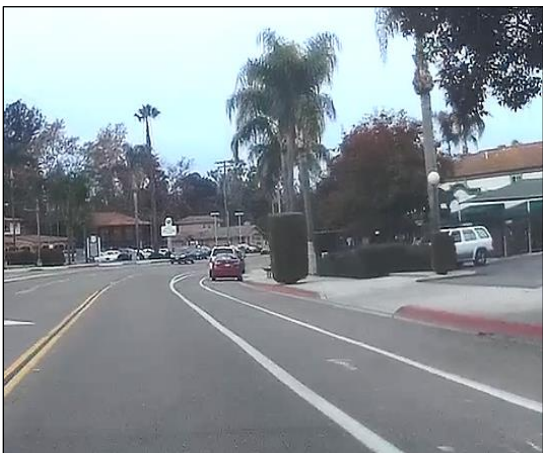
Bicycle lane east of Williamston Drive
