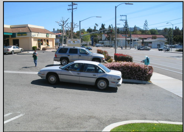
Entry throat is too short, resulting in the need for drivers to make decisions too soon after exiting the street. This slows drivers down, potentially causing traffic back ups on the arterial and endangering pedestrians.
