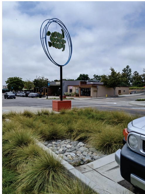
Figure 1. Bioretention basin on Main Street in Vista
