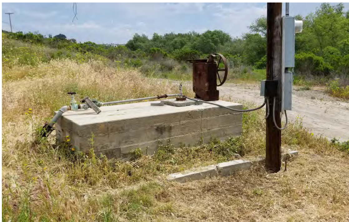
Photograph 7. Overview of CA-SDI-5652 water pump feature, facing east
