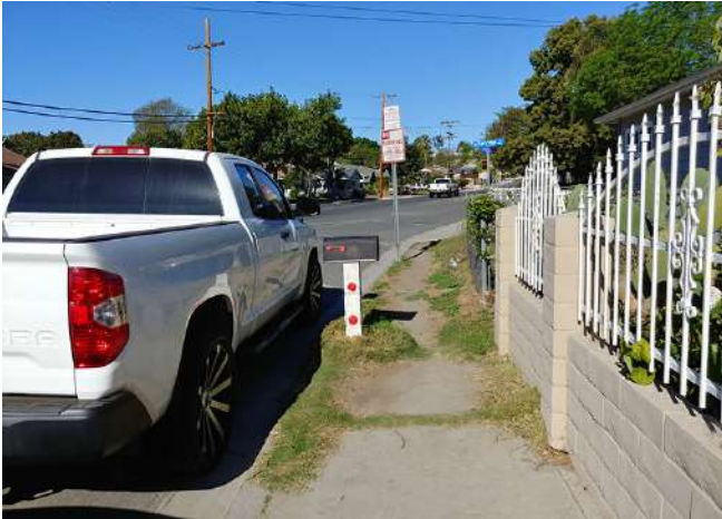
Disconnected sidewalks and delineated foot paths/desire lines
