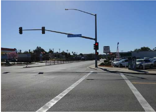
Median fence to deter midblock crossings
