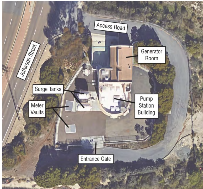
Figure 3-6. Existing Buena Vista Pump Station
