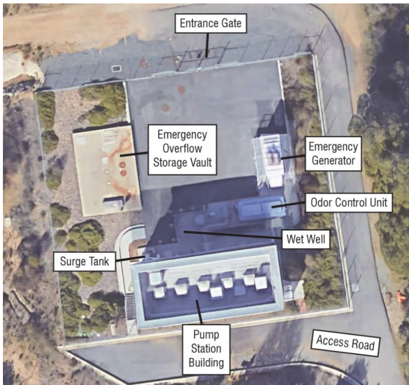
Figure 3-5. Existing Buena Creek Pump Station
