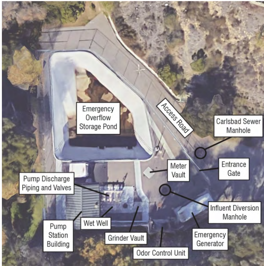
Figure 3-4. Existing Raceway Pump Station
